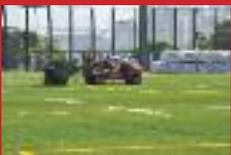
9. Infilling of the Eco-cool rubber or SBR rubber layers.
